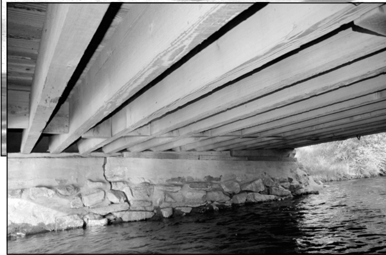
TROUBLED BRIDGE OVER WATER: Above, the closed-off bridge at road's end in Mineral King. Left, the underside where some supports are rotted.
