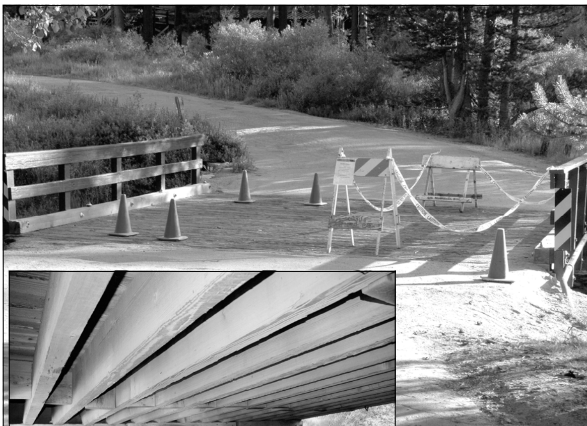
TROUBLED BRIDGE OVER WATER: Above, the closed-off bridge at road's end in Mineral King. Left, the underside where some supports are rotted.
